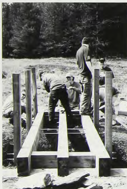
Volunteers building a bridge for the Schiehallion path. Photo by Alison McGachy
