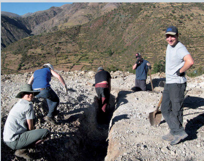
Digging the foundations at Sanayca
